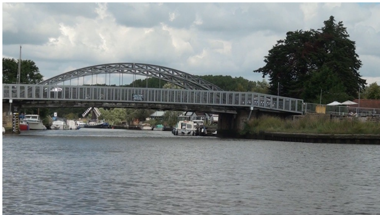
St. Olaves Bridge
